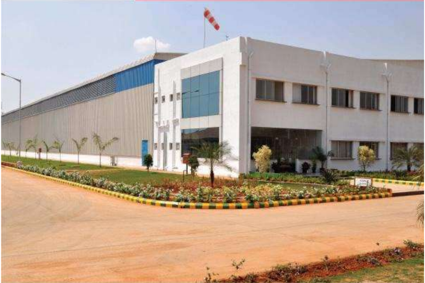
State-of-the-art plant of Wienerberger Brick Industry Pvt. Ltd., Kunjal, Bangalore, India.
